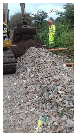
Access to centre of bund / hibernacula by drainage pipes, inserted every few metres. Compacting of the top soil and bund structure completion.
