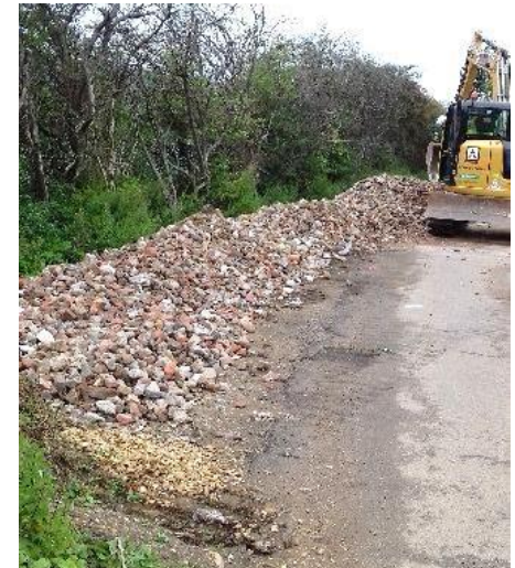
Rubble core of bund laid down by digger
