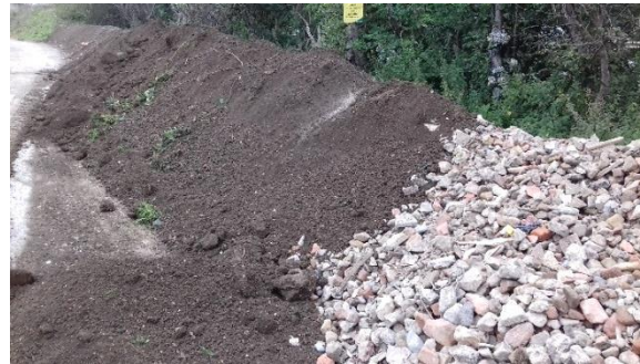
Top soil layer covering and insulating the heart of the bund.
