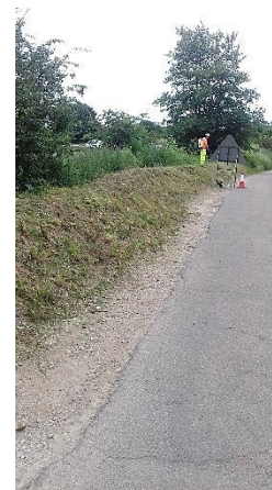
Strimming of self-set vegetation. Bund after raking and seeding with wildflower seed.
