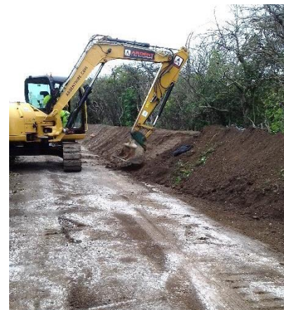
Access to centre of bund / hibernacula by drainage pipes, inserted every few metres. Compacting of the top soil and bund structure completion.
