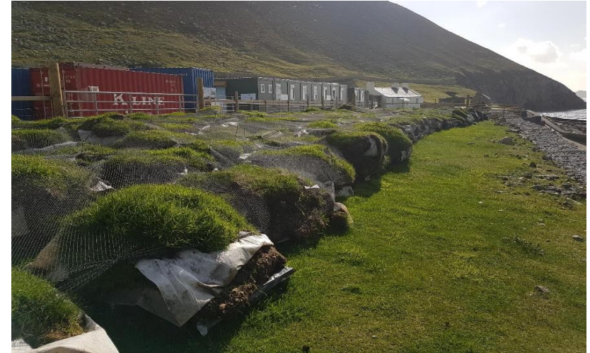
Turf stored on pallets and fenced off from Soay sheep for the reuse on the roofs of the new building.
