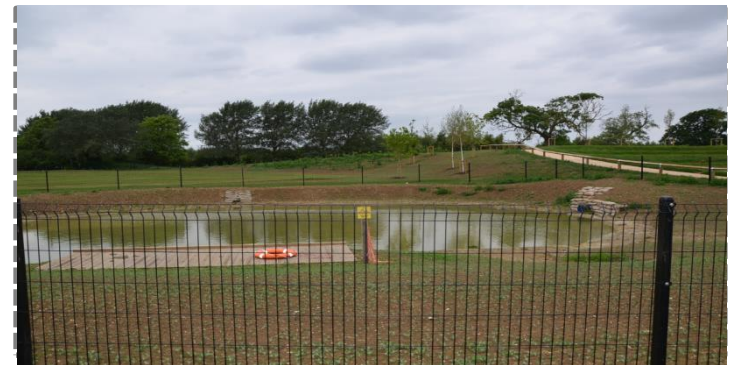
Credit: Andrew Gladwin, Willmott Dixon Permeable pond with drainage feeding into it
