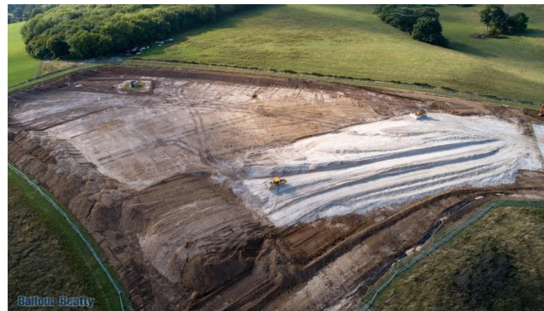
Placement & Compaction of chalk from main site to form the calcareous sub-base - 13/08/2018
