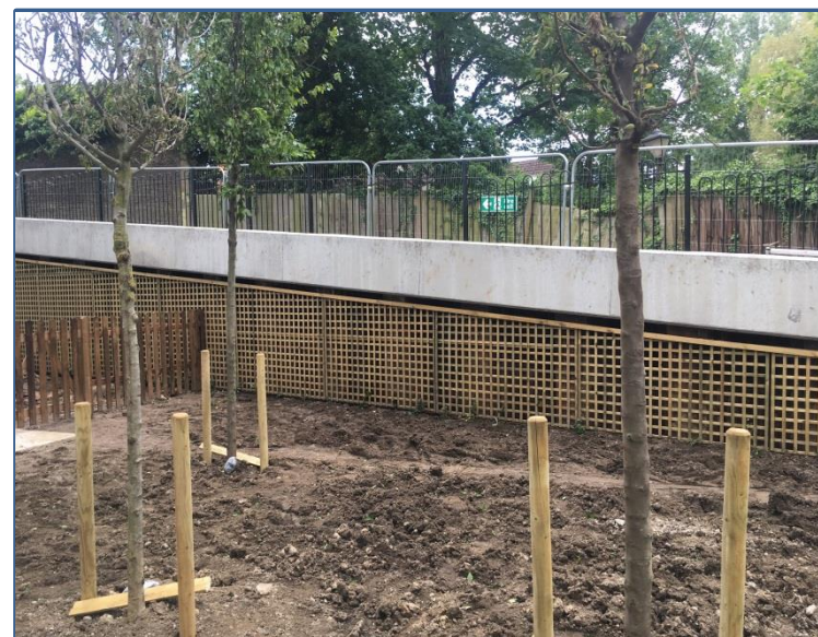
20 metres of trellis fencing living wall along sheet piling.
