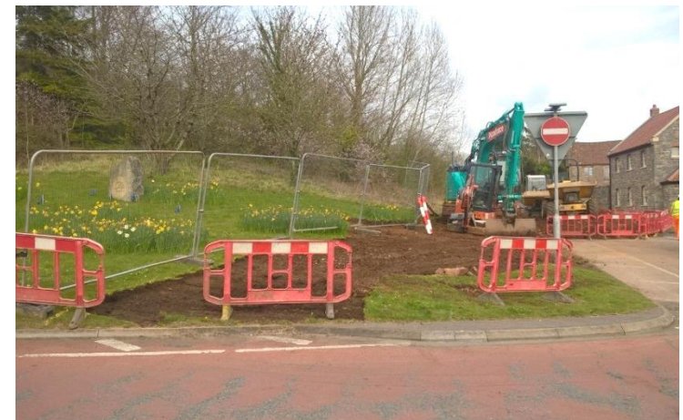
View of stripped area where SSSM would be laid, reduced working space to avoid unnecessary disturbance
