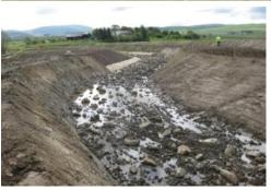
soil structure restoration channel for low flow Willow whips planted close to the waters edge will stabilize banks, interact with flow and provide leaf-litter to the stream bed
