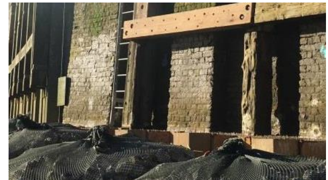
Above: 1 Coldharbour lane timber fenders and Kyowa bags installed, predrilled holes visible on the fenders.
