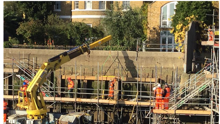
Installation of the timber fenders:
