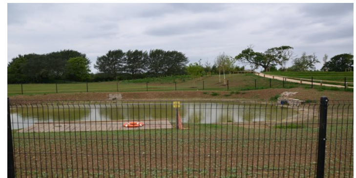
Permeable pond with drainage feeding into it Credit: Andrew Gladwin, Willmott Dixon
